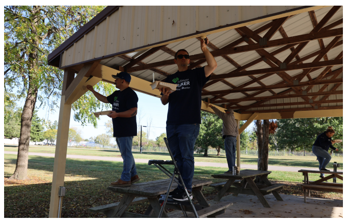
Painting shelter houses at Johnson County Park.
