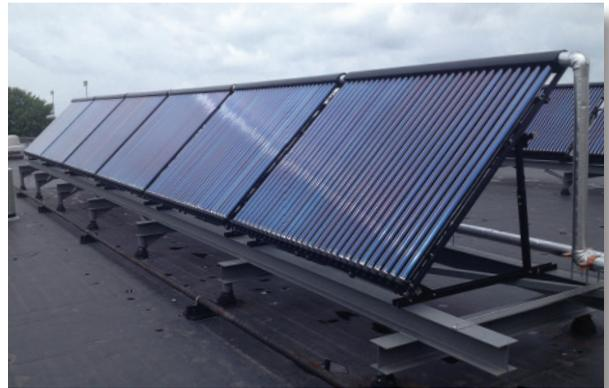
supplementing an existing water heating source. The systems have a 25-year service life and can reduce carbon dioxide by up to two tons per year.
